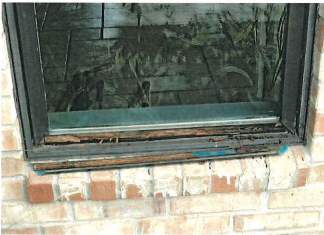
The image above shows a window that needs its sash and sill replaced. The entire window does not need replacing.
