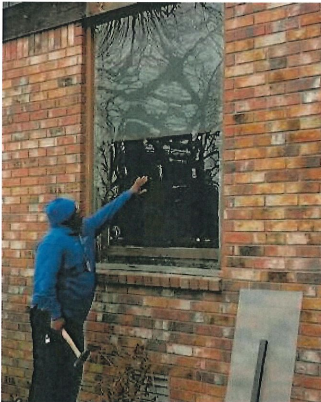
Clear polycarbonate sheeting board is the preferred window covering for existing windows in downtown Moberly.
